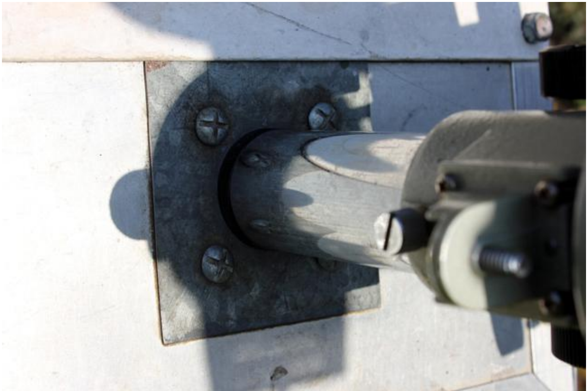
Figure 3. Additional steel sheet around the end of the draw tube.
